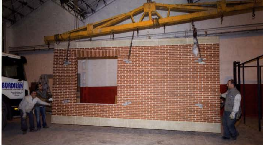
Installation of partition walls
