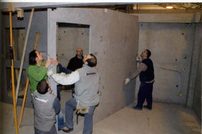
Module with installed underfloor heating system, prior to screeding
