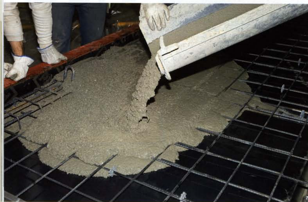
Construction of the concrete base, using self compacting concrete
